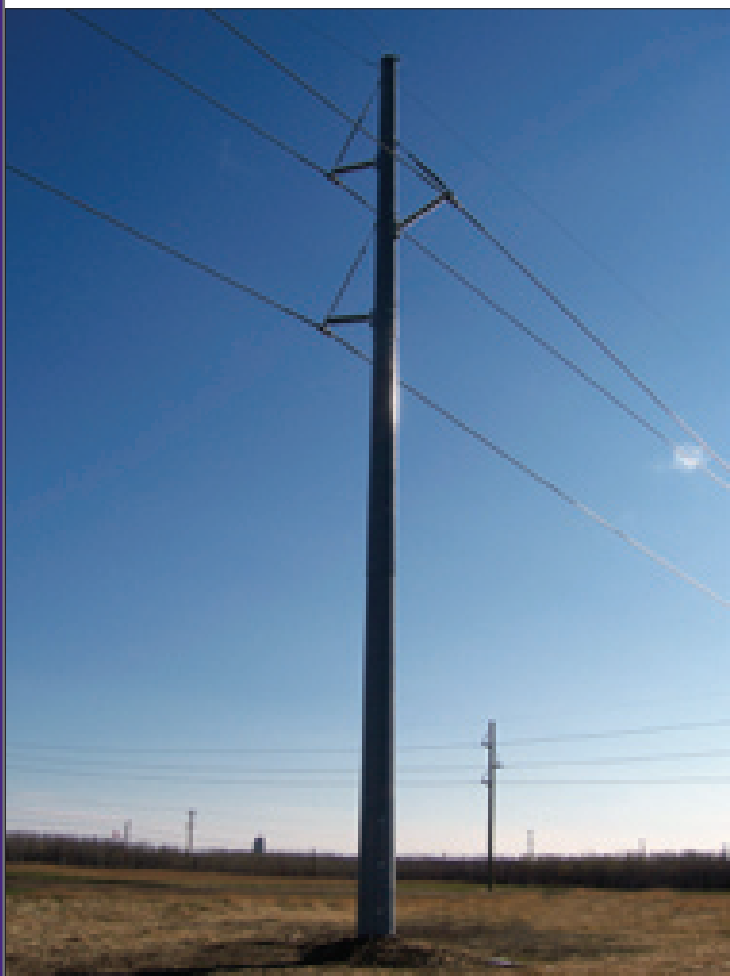
RS's installed utility pole. Photo credit: Resin Systems Inc.
